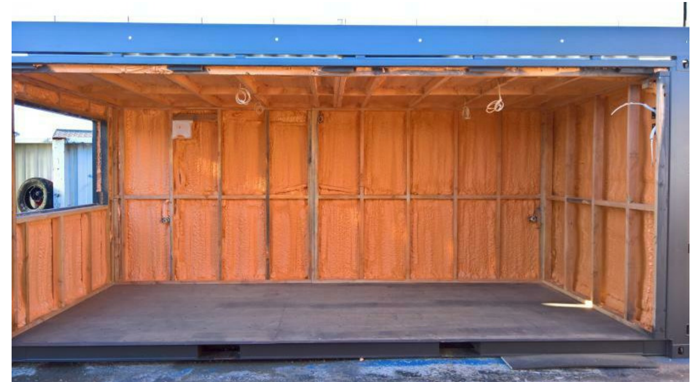
SPRAY FOAM COMPLETE
