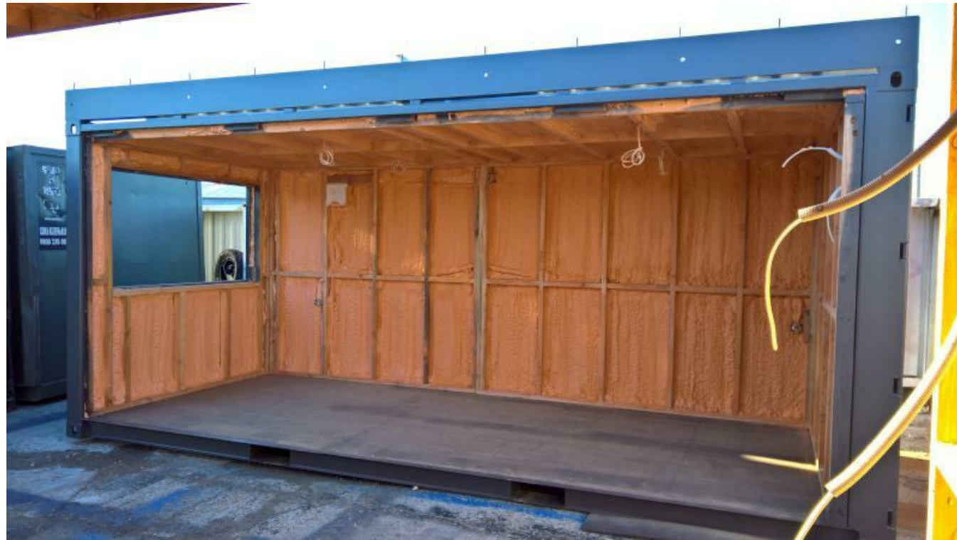
SPRAY FOAM COMPLETE
