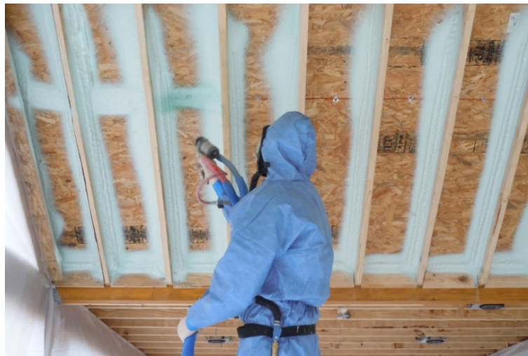
Figure 7: HEATLOK HFO applied to underside of cathedral roof/ceiling or deck system
