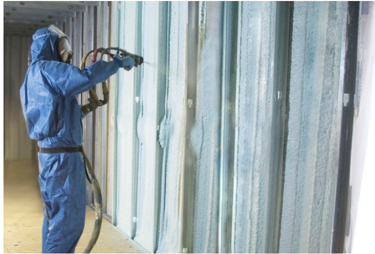
Figure 6: HEATLOK HFO applied between wall studs.
