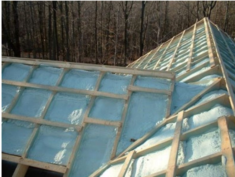
Figure 2: HEATLOK HFO applied to a roof/ceiling prior to roofing
