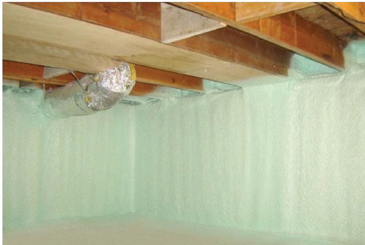
Figure 3: HEATLOK HFO applied to under floor sub wall
