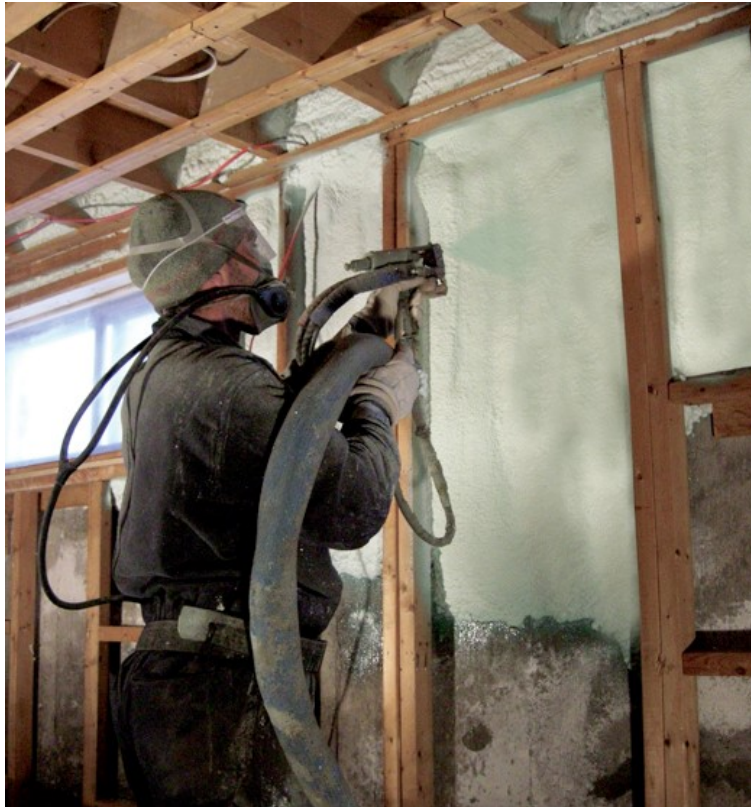
Figure 4: HEATLOK HFO applied to external facing wall with a Rigid Air Barrier installed.
