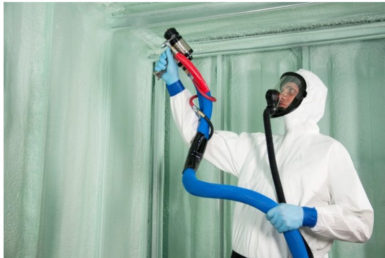
Figure 1: HEATLOK HFO applied to wall and ceiling
